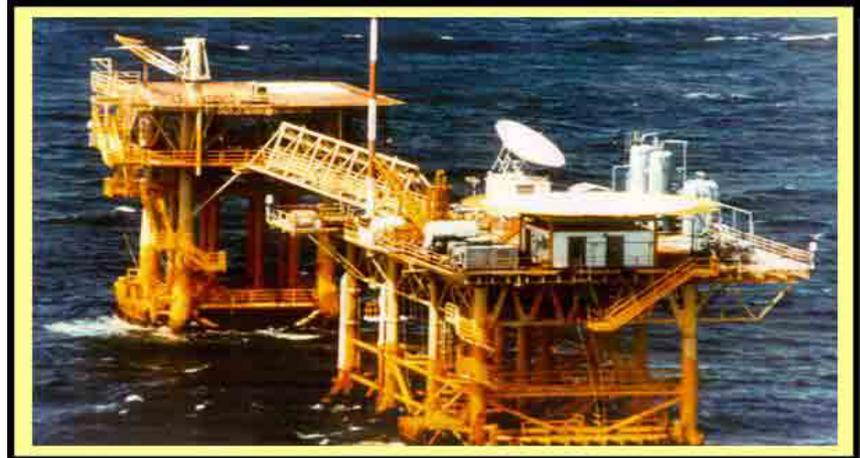
***“...constructed by Conoco in 1984, with 120 mmcf/day capacity. Refurbished in 2003 to handle current production.”***
